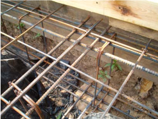
reinforcing steel in a perimeter stiffening beam of a slab-on-ground foundation
