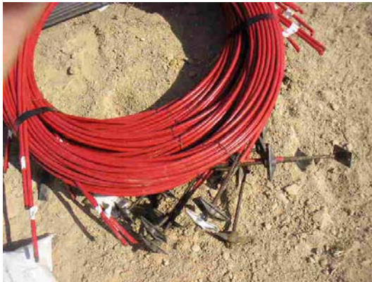
this is a bundle of post-tensioning cables as they are delivered to the site
